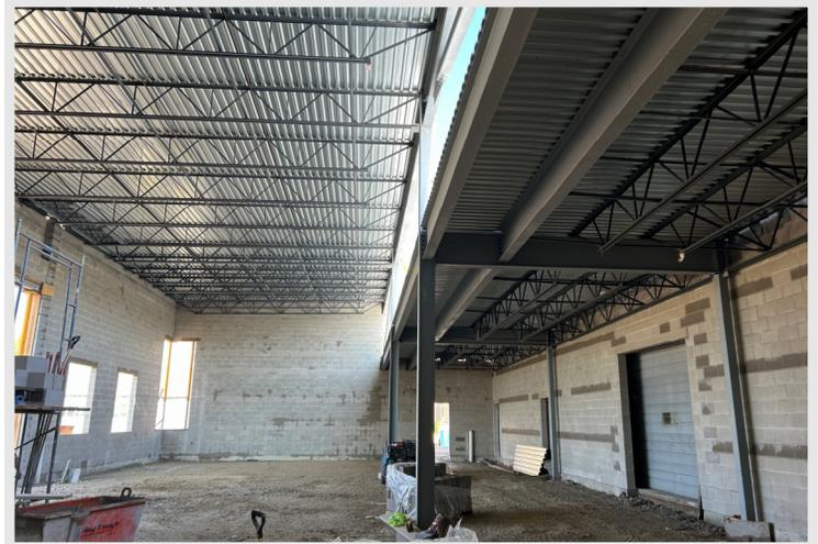
Findorff structural steel crews have completed the main steel structure at the Skills Lab Addition. Detailing work will continue the next few days.
